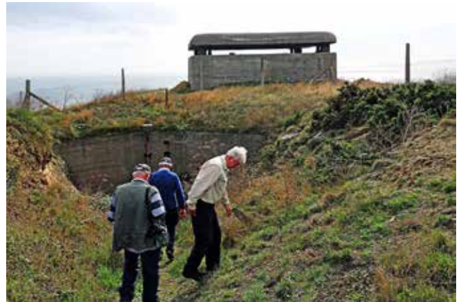
Approaching the command post of Batterie Generaloberst Dollmann on the cliff top overlooking Gull Rock. This is a distinctive two-level semi-sunken bunker with a square roof raised on pillars above the rangefinder position. This was used by Guernsey Civil Defence as a nuclear monitoring post until the 1980s when it was abandoned following persistent vandalism and a new post was opened in one of the island's four telephone network junction bunkers nearby at Torteval
